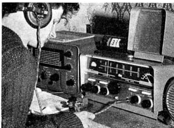
G3MZX operating GD6UW during the Cambridge University Wireless Society's expedition to the Isle of Man at the beginning of April. The Hammarlund HX50 s.s.b. transmitter is on the left of the photograph and the K.W. Electronics KW77 receiver on the right.
